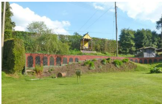
The completed project (left side)
