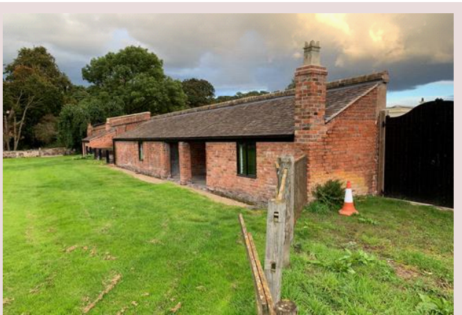
Refurbished back sheds
