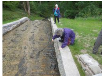
Daphne Capps supervises Nicky Lipscombe as she clears a spillway.
